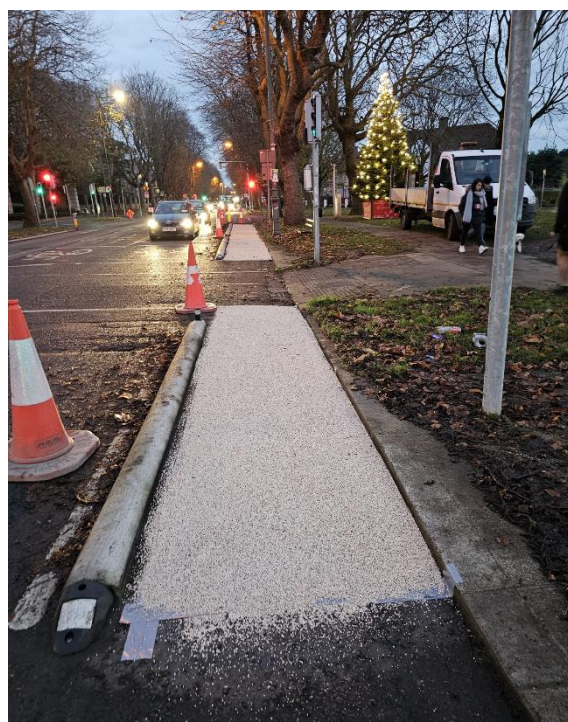
Last of coloured surfacing being applied to Griffith Avenue
